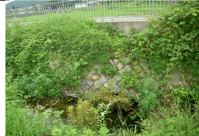
護岸の破損
