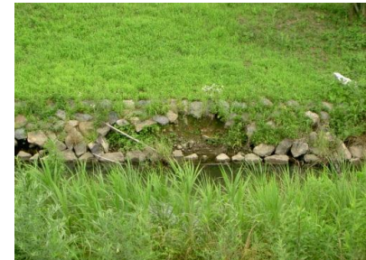
護岸の破損
