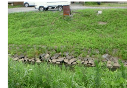
護岸の破損
