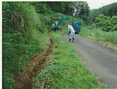
側溝掘削100m
