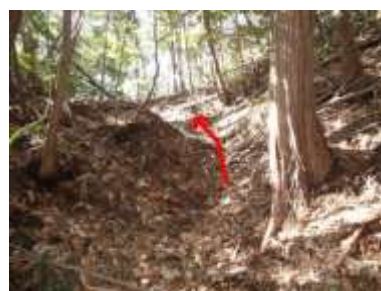
(施工前)林内歩道
